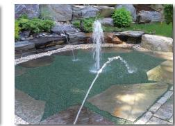
A soft version of Porous Pave using all rubber chips and a softer binder
